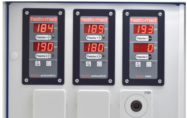
Overview at a glance: External display and control unit for oxygen and compressed gas cylinders.
